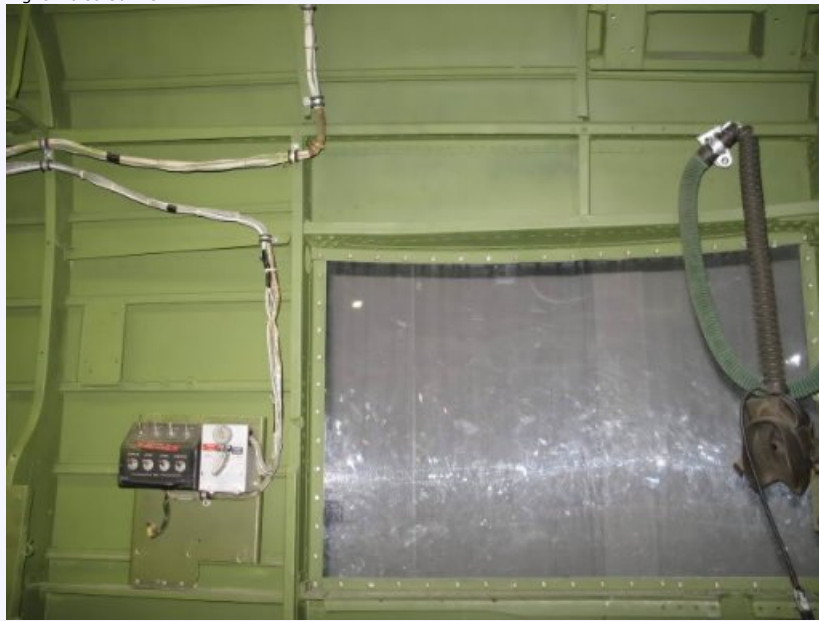
Right Escape Hatch
